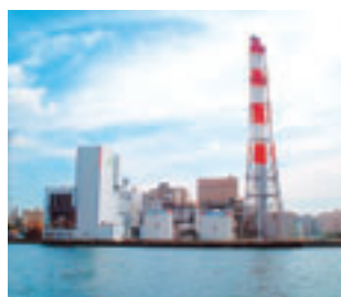
Fuel for No. 3 generation unit at the Kawasaki Thermal Power Plant was completely switched from kerosene to natural gas in June 2006.
