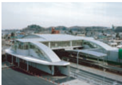
Hakonegasaki Station on the Hachiko Line, an open-plan structure with a dome-shaped roof and many glass panels.
