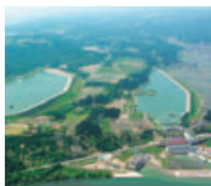
The Shinanogawa Hydroelectric Power Station restarted full-scale operation after earthquake damage was repaired.
