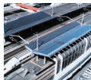
PV panels installed on the roof of the Shinkansen platforms at Takasaki Station.
