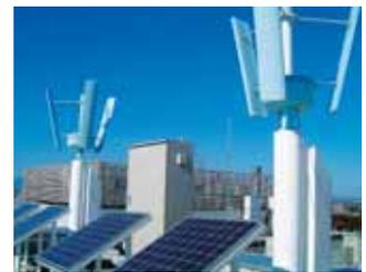
Wind power generator on the roof of Kokubunji L Terminal Building. A display screen inside the building indicates how much power is being generated at any given time.
