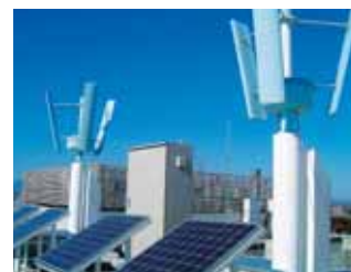
Wind power generator on the roof of Kokubunji L Terminal Building. A display screen inside the building indicates how much power is being generated at any given time.
