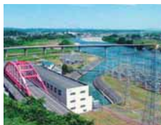
Shinanogawa Power Station, damaged by earthquake. Repairs are underway.
