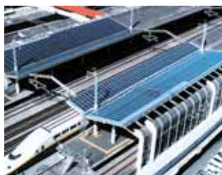
PV panels on roof of the Shinkansen platform at Takasaki station provide electricity for lighting and air conditioning.
