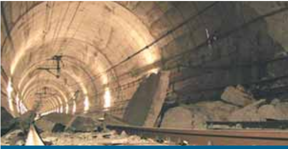
Scene of the Joetsu Shinkansen Uonuma Tunnel, about 2.4 km from the tunnel entrance. The earthquake damage was far greater than generally expected.
