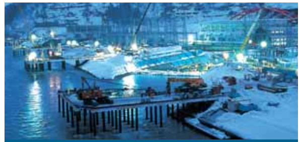
The Shinano River Hydraulic Power Plant, operated by JR East, was damaged by the earthquake. Amid a heavy snowfall, repair work continued day and night to get the water flowing again as soon as possible.
