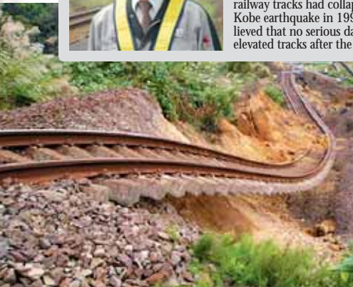
Many sections of conventional line tracks were also damaged. Efforts to inspect the damage were conducted while taking care to avoid secondary disasters.
