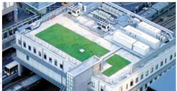
View of rooftop of the JR East Shinjuku Nambu Gengyo Office, the first of JRC's rooftop greenery projects.
