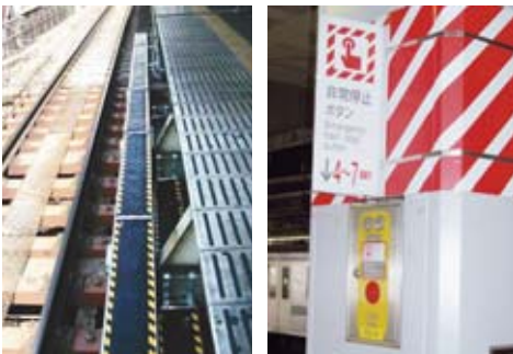
We are installing a variety of safety systems on station platforms, including mats that detect when a person has fallen upon the tracks (left) and emergency stop switches (right).
