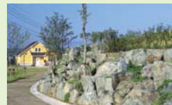
Natural stone walls and greenways paved with pumice stones
