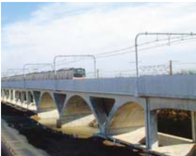
The bridge between Minamikoshigaya and Yoshikawa Stations has v-shaped bridge supports to harmonize with the surrounding environment
