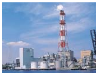
Kawasaki Thermoelectric Power Plant; aging power-generating unit 4 is scheduled for upgrade to highly efficient high-output combined-cycle power-generating units.
