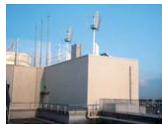
Wind power generator on the roof of Kokubunji L Terminal Building. The amount of power generated at any given time can be checked on a monitor screen inside the building.
