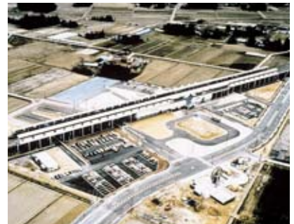
A Park & Ride at Kurikoma Kogen Station on the Tohoku Shinkansen
