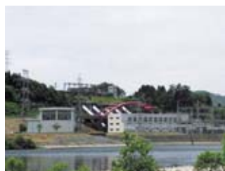
Three plants, Senju, Ojiya and Shinojiya, make up the Shinanogawa Power Station with a total output of 450,000 kW.
