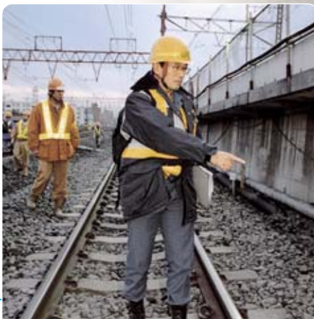
▶ Final checks are carried out thoroughly.
