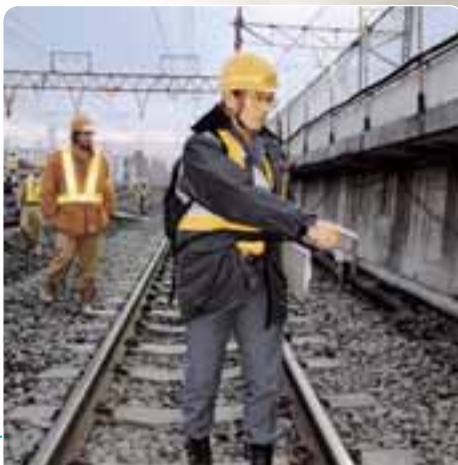
▶ Final checks are carried out thoroughly.
