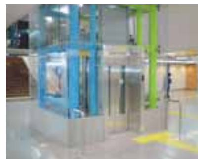
We are installing elevators to eliminate barriers to mobility.
