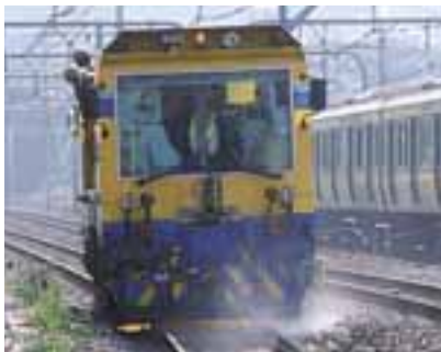
Rail alignment vehicle trims and flattens rails between Iidabashi and Ichikawa Stations on the Chuo/Sobu Line.
