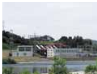
Three plants, Senju, Ojiya and Shinojiya, make up the Shinanogawa Power Station with a total output of 450,000 kW.
