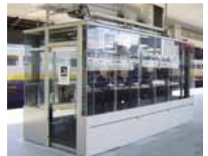
In order to promote prohibitions on smoking, completely-enclosed rooms with exhaust facilities have been installed as smoking areas on some Shinkansen platforms.
