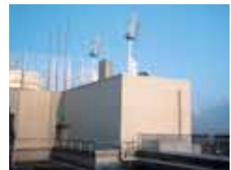
Wind power generator on the roof of Kokubunji L Terminal Building. The amount of power generated at any given time can be checked on a monitor screen inside the building.
