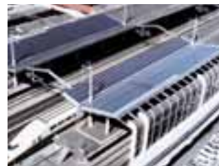
The number of solar panels on the Shinkansen platforms at Takasaki Station has been doubled
