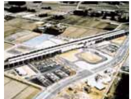
A Park & Ride at Kurikoma Kogen Station on the Tohoku Shinkansen
