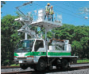
Rail-based heavy machinery makes aerial work safer
