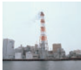
Working to reduce CO 2 emissions from thermal power plants
