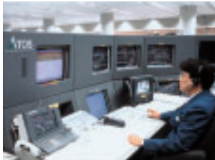
The ATOS command center provides centralized control for all designated trains
