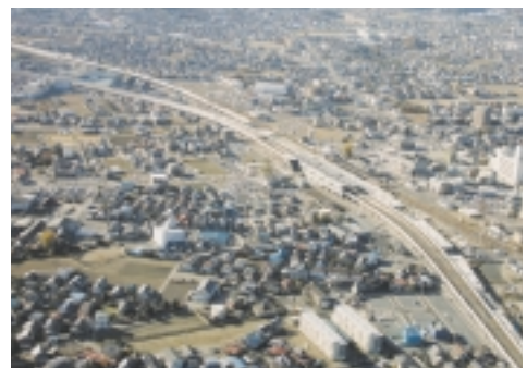
Continuous overhead crossing
