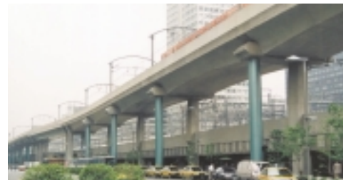
Viaducts in the vicinity of Tokyo Station on the Chuo Line
