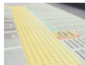
Raised tiles for guiding visually impaired persons
