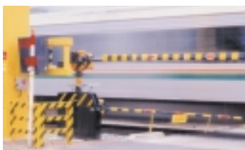
Two stage type crossing gates
