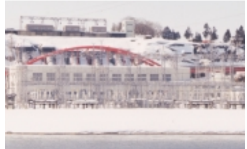
Shinano River Power Plant
