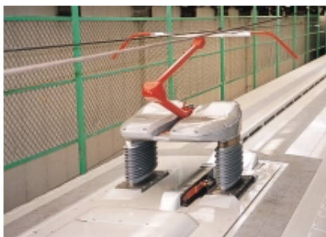
A new single-arm pantograph and insulator
