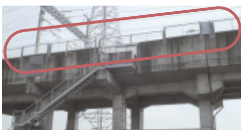
Soundproof walls of transparent plates
