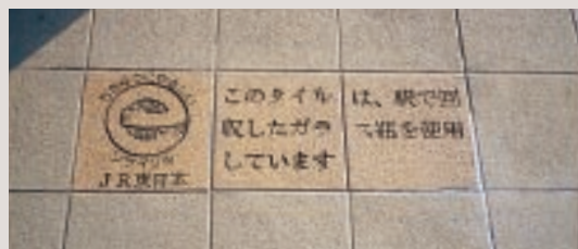
Recycled paving tiles made from glass bottles (platform at Hitachi-no-Ushiku Station)
