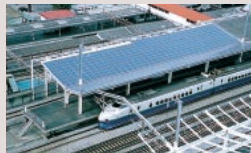
Photovoltaic generator units
