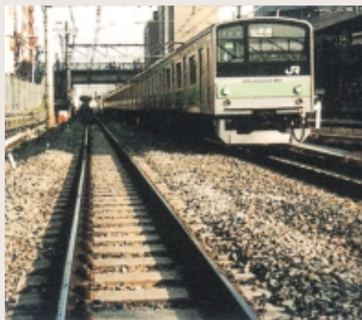
"TC-type low-maintenance roadbed," introduced to reduce labor spent in maintenance work
