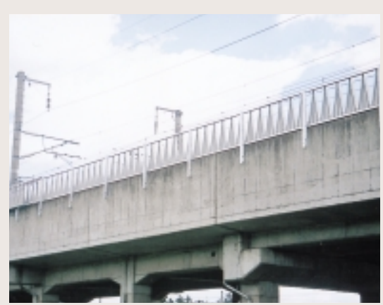
The Dancette noise-insulation structure, which cancels noise through interference.
