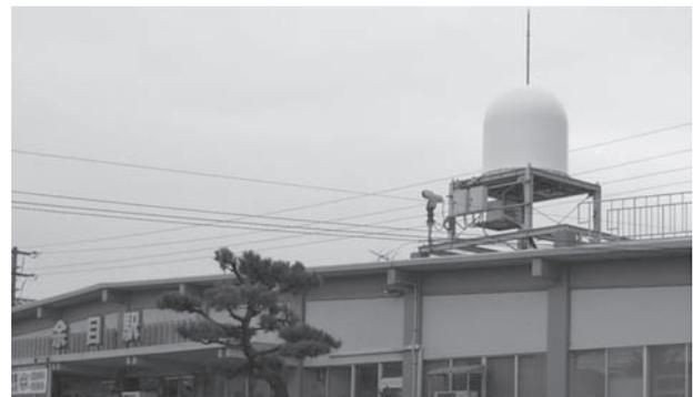
Fig. 1 Doppler Weather Radar on Roof of Amarume Station
