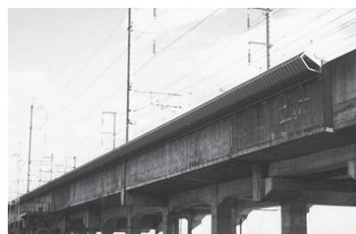
Fig. 1 Interference-type Noise Reduction Device
