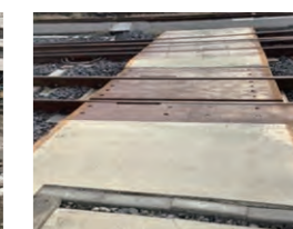
Walkway maintenance (prevention of falls)
