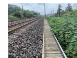
Construction surface improvement (prevention of struck-by accidents)
