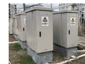
Cubicle installation (prevention of electrocution)
