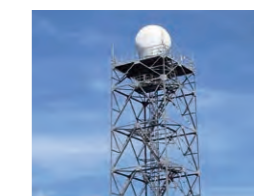
Countermeasures against gusts using Doppler radar
