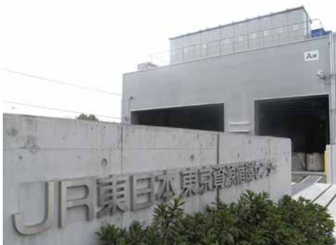
JR East Tokyo Materials Recycling Center
