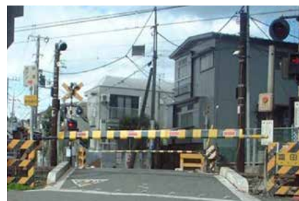
A large crossing gate
