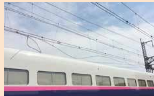
April 29, 2015 Transport disrupted by cut overhead contact line at Koriyama station on the Tohoku Shinkansen route
