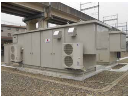
Kuki substation power storage system
