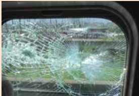
Aug. 9, 2015 Broken window pane on a Tohoku Shinkansen train
