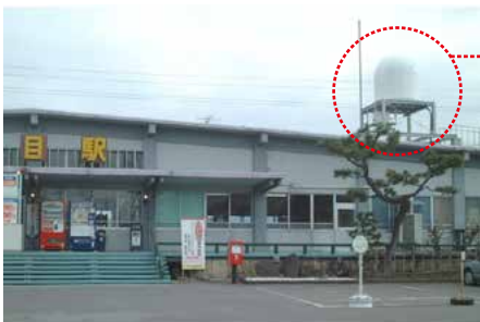
Doppler radar installed on the roof of Amarume Station on the Uetsu Main Line
