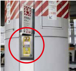
Emergency stop buttons on platforms
