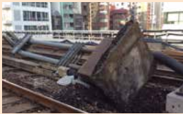
April 12, 2015 Electric post collapsed between Kanda and Akihabara on the Yamanote line (serious incident)
