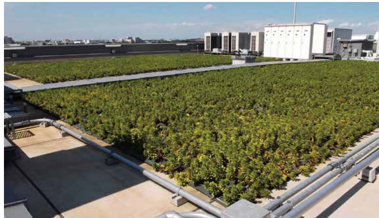
Rooftop greenery at the Chiba branch building
