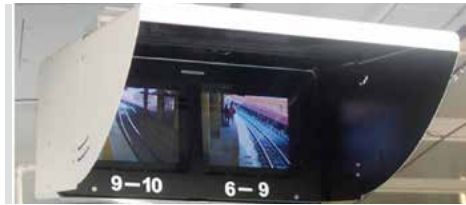
ITV for station platforms and concourses
