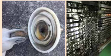
March 15, 2016 Transport disrupted by breakdown of electrical equipment at Kagohara station on the Takasaki line
