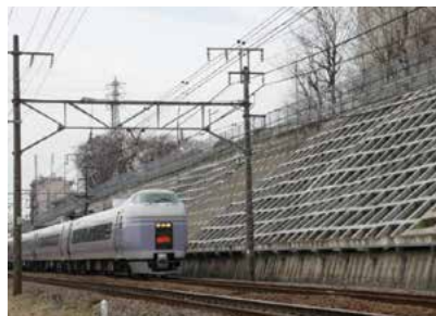
Cutting slope protection (spray frame work)
